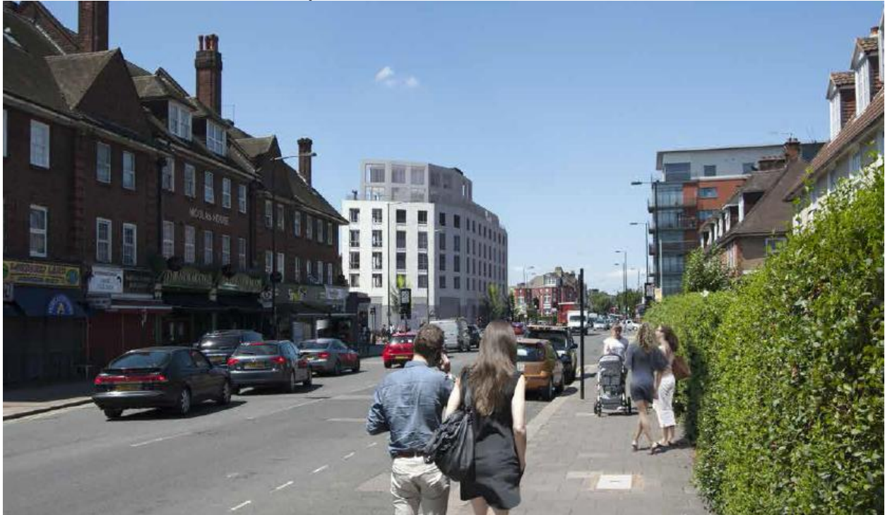
View from east on Lordship Lane
