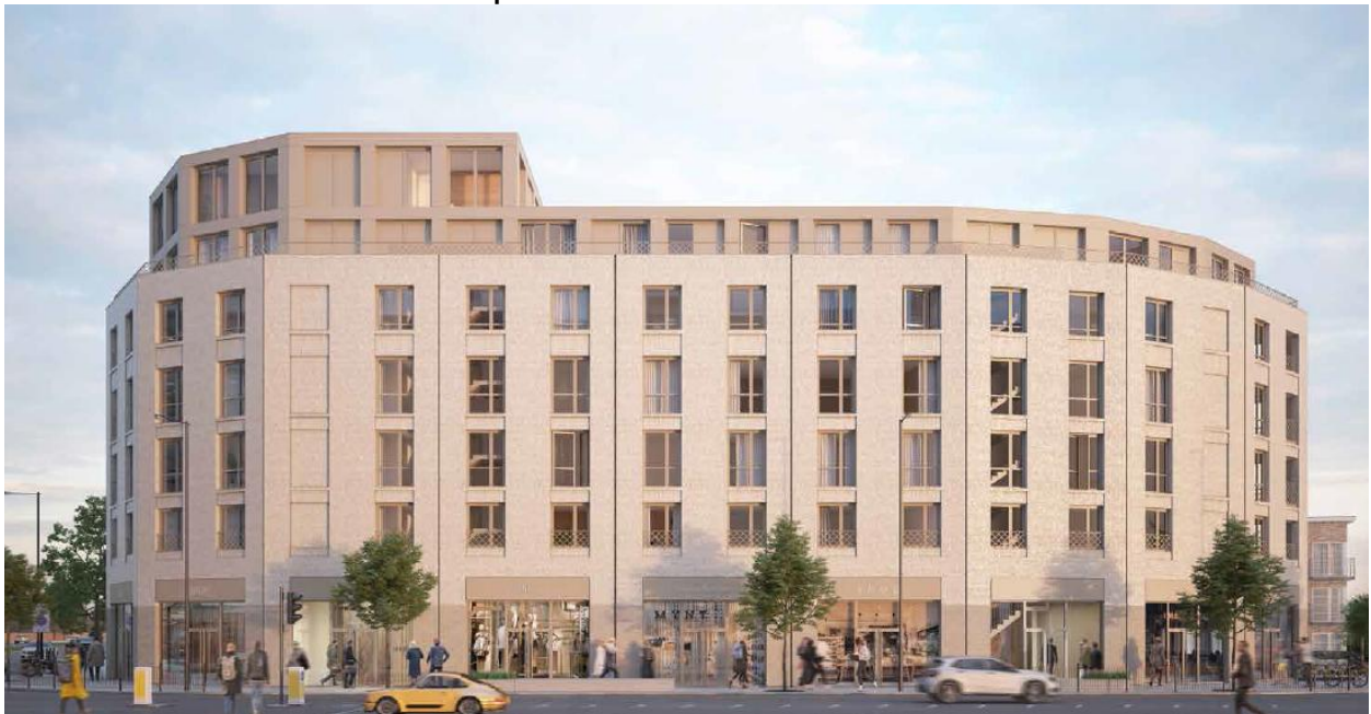
View from north on Lordship Lane
