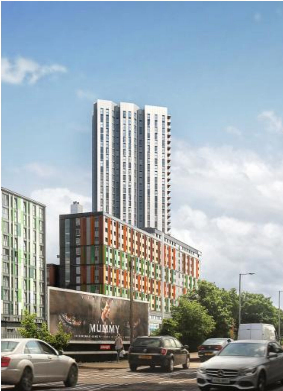
View of Building from North on Ashley Road
