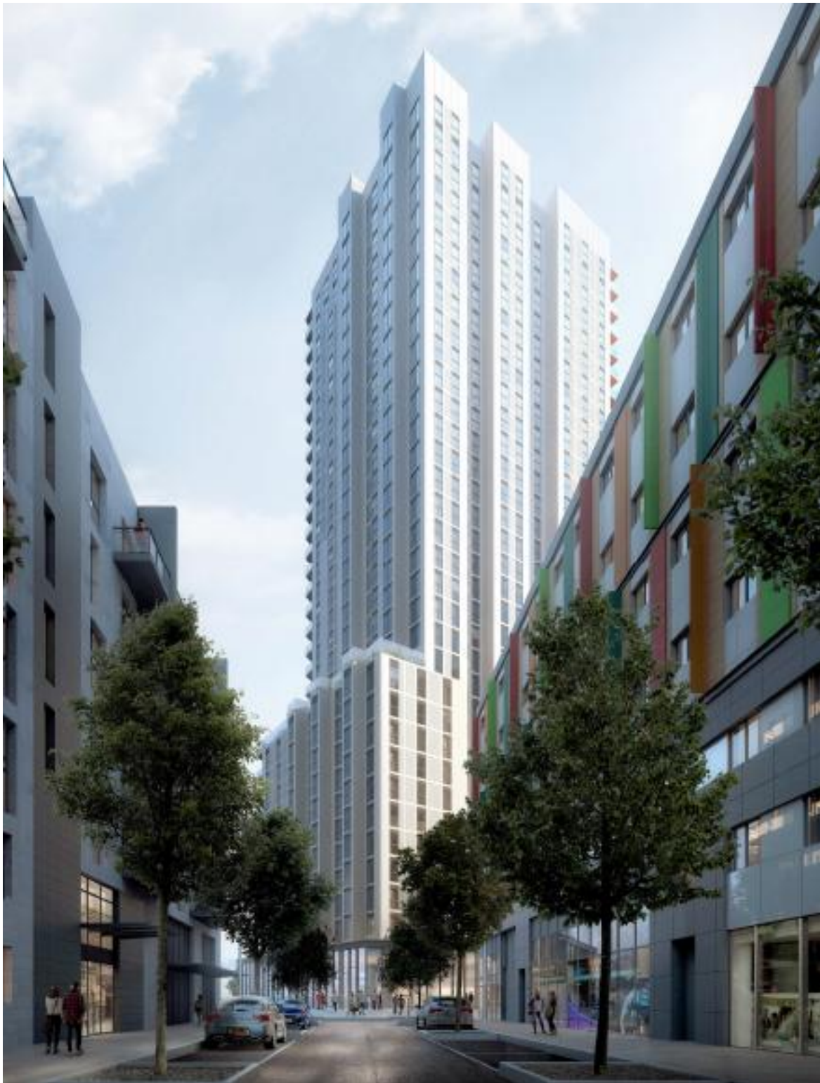
View of Building from North on Lebus Street
